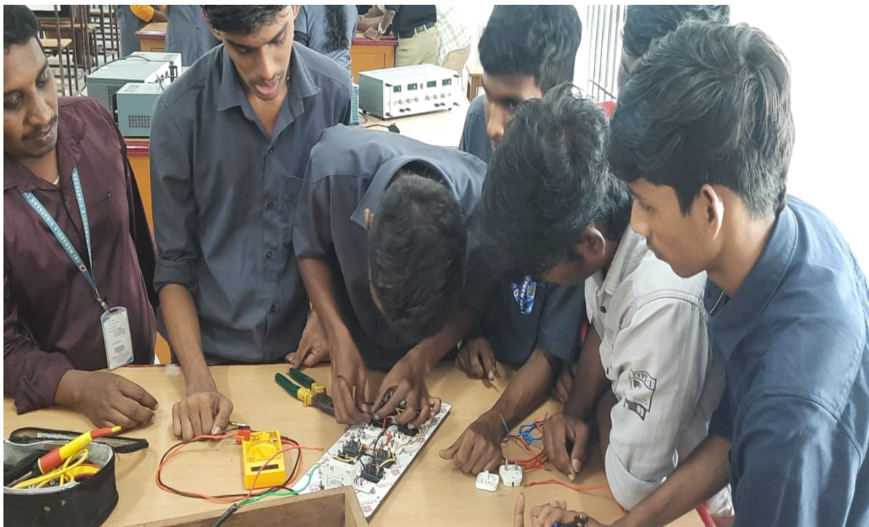
Students Actively connected the switch board wiring in a practical manner under the Guidance of Mr.J.Muruganandham.
